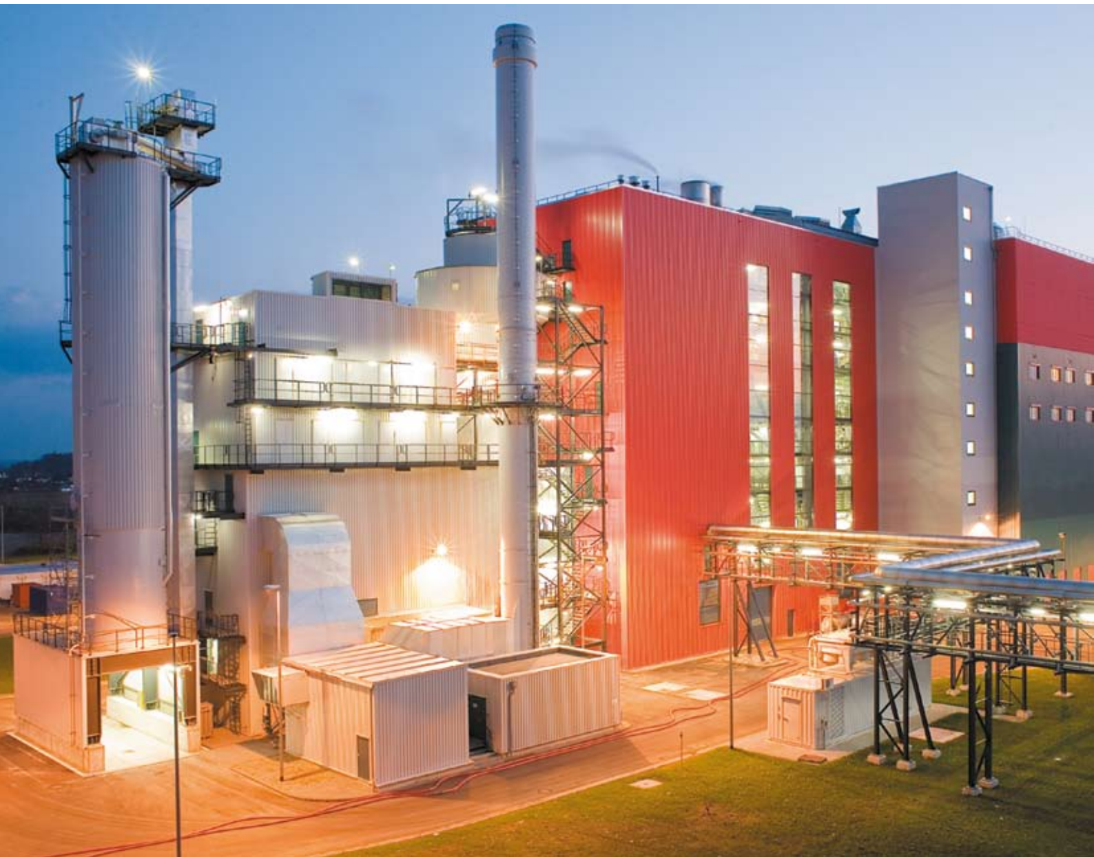
E.ON Energy from Waste plant, Premnitz
